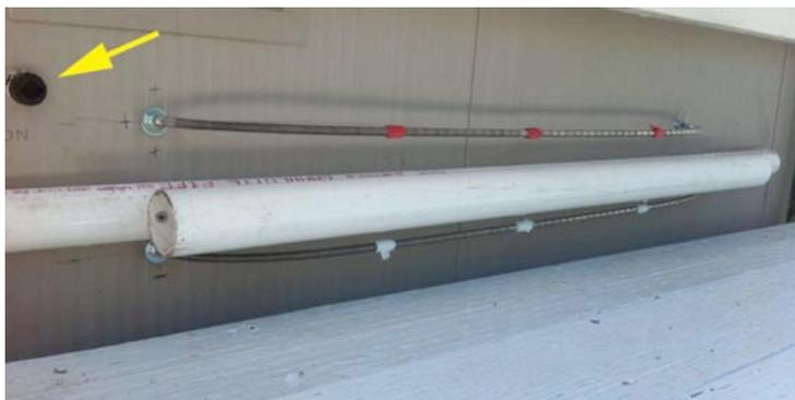
Two power terminals separated by two PVC pipes. Insert key into the black hole marked by the yellow arrow in the photo above.
