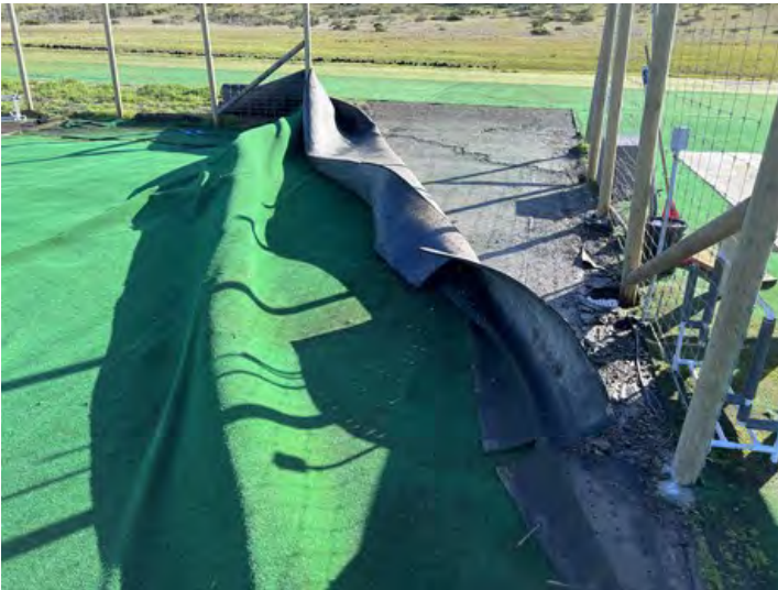
The wet pit entrance was in a rough shape!
